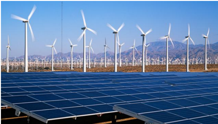
Figure 3: A typical wind power generation [9].
