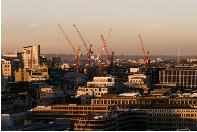
Figure 5: A typical construction site [8].
