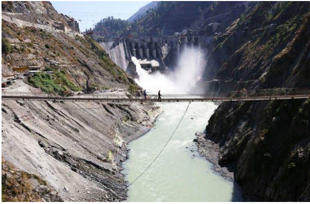
Baglihar Dam on the Chenab River, Source -Amit Gupta/Reuters
