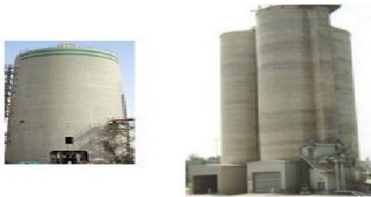
Figure 2: Fly Ash Storage silo
