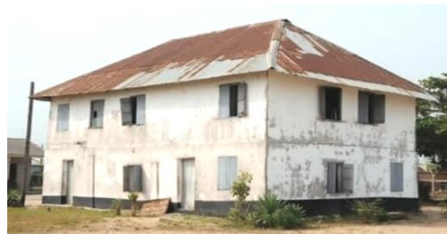
Plate 3: A two storey building Badagry, Lagos, Nigeria. (The second in Nigeria in terms of age)
