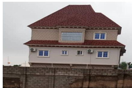
Plate 2: A modern three storey building in Asokoro Abuja, Nigeria with the semblance style of ancient Odogo building.
