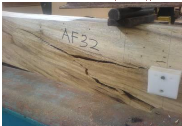
Figure 4 Typical cracking of an AF beam
