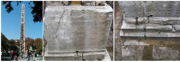
Fig 2: The base of an Egyptian obelisk that illustrating the stone layers of the base as a method of base isolation.
